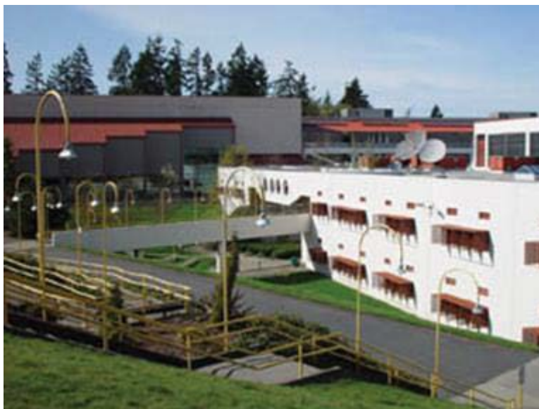
White building, east building.
