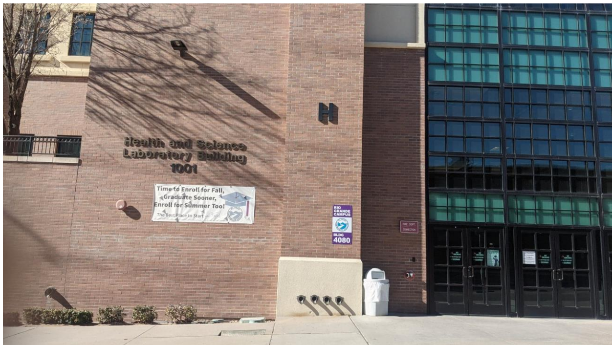
Pictured above is the Health and Sciences Laboratory Building #4080 (H-Building)
