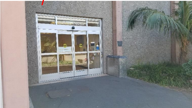
Enter from the back of the building.
